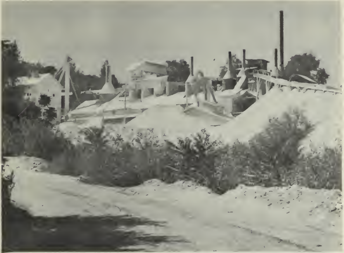
A, PLANT OF U. S. LIME PRODUCTS CORPORATION Sonora, Tuolumne County. Limestone used here is from Carboniferous Calaveras formation. Olaf P. Jenkins, photography, 1948.
